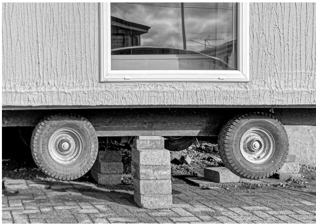
One half of a double-chalet awaiting settlework and boxing. © Graham Skeate
