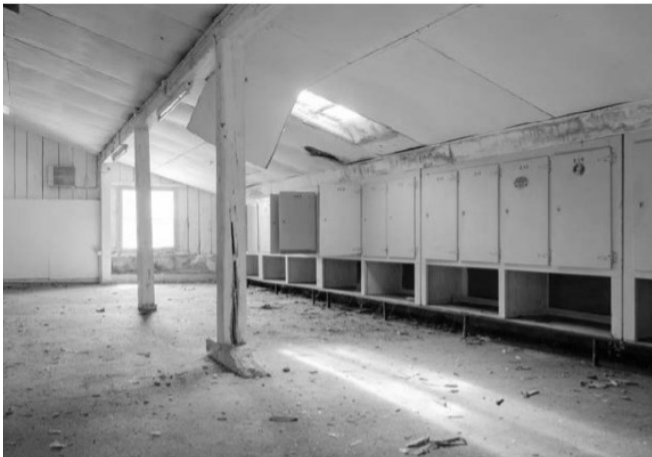
A row of windows in the attic as architectural evidence of home-based work in the watch industry. © Florian Eitel, 2023
